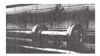
A magnetic unit installed at GKN's technology centre treats water to prevent scale. It contains four permanent bar magnets and constrictions in the pipe make the flow of water or other fluids through it turbulent. This, however, has a secondary effect when it comes to preventing scale. The unit alters the way in which crystals form, changing their size and ability to form scale
