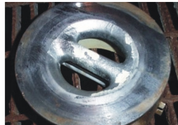
No Scale Build Up After 8 Months With MFC's Installed
