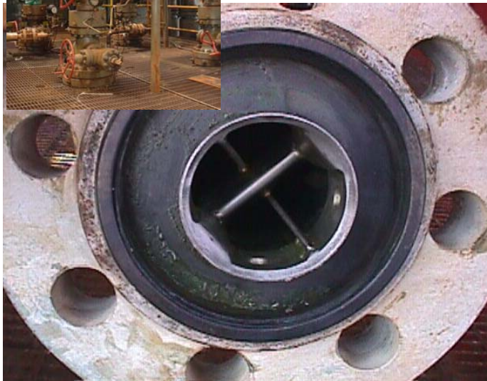
Scale-X ® magnetic fluid conditioner installed in BGEPIIL Mumbai well head piping
